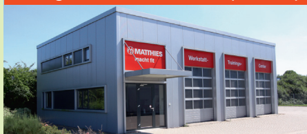
Trainings-Center ROTENBURG (Flexwerk)
